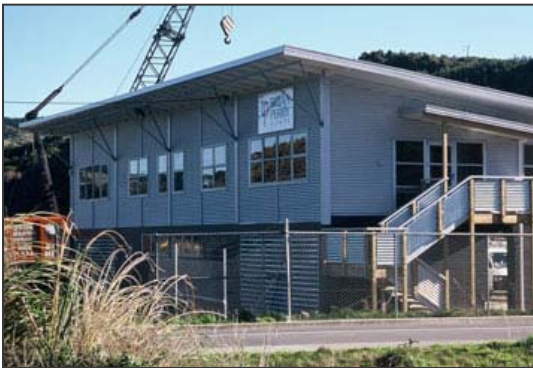
Figure 2: Elevated industrial building 14
