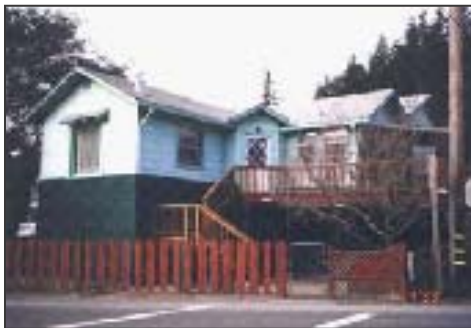
Figure 9 & 10: House before and after elevation 23
