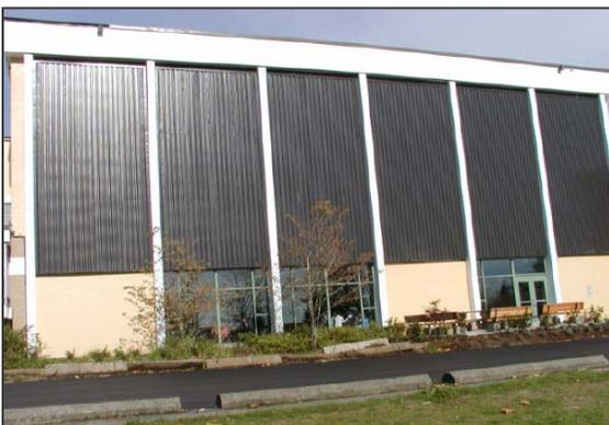
Figure 6: A 214 m<sup>2</sup> (2300 ft<sup>2</sup>) SolarWall installed on Centennial School's gym in Coquitlam provides fresh air at a rate of 6,000 CFM (Source: SolarWall)
