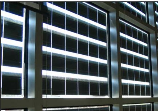
Figures 1 & 2: The 12.8 kW Building Integrated Photovoltaic array incorporated into the curtain glazing of Red River College’s Princess Street Campus (The photo on the right shows this system from the inside).
