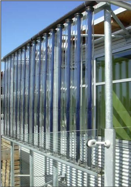
Figure 4: Solar tubes at the City of White Rock's Green Operations Building
