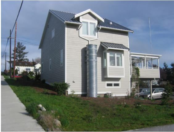
Figure 4: This cistern collects rainwater from the roof for non-potable domestic uses.
